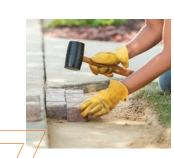
Use a rubber mallet to tap your pavers into the sand to level and make as snug of a fit as possible. Continue the process all the way to street.
