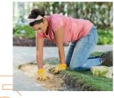
After the base gravel is even and level, add in around 1"-2" of paver sand (not playground sand as it doesn't compact as well as a paver sand layer). Use tamper to compact and level the sand.
