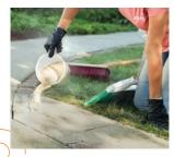
Lay down polymeric sand. Use push broom to push into seams and wet down with hose.
