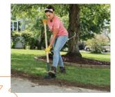
Use a shovel to roughly dig and level out. Over excavate so it's at least 6" wider than the paver design. Compact and level off the dirt.
