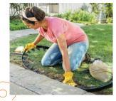
The outside pavers should be locked into space with an edge. You can do this by using a plastic paver edge with stakes.
